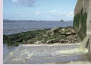
SEWAGE OUTFALL, GARSTON
