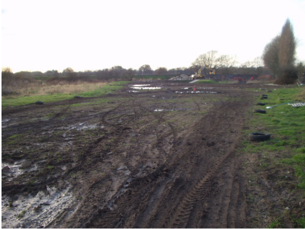
Mersey Vale site before work began
