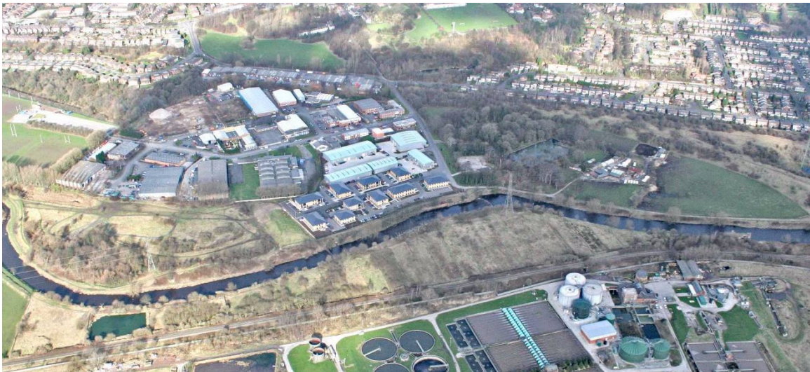
Mersey Vale site before work began
